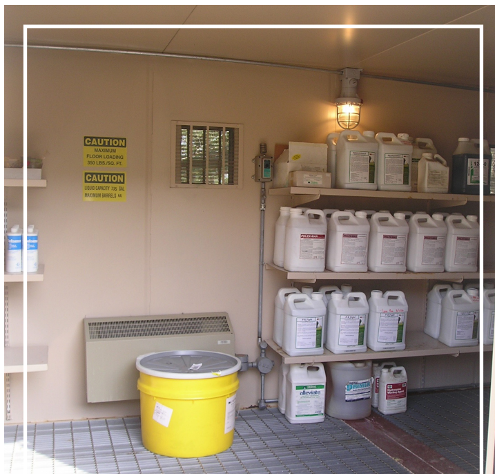
Modern chemical storage structures with secondary containment provide a safe way to store chemicals.
